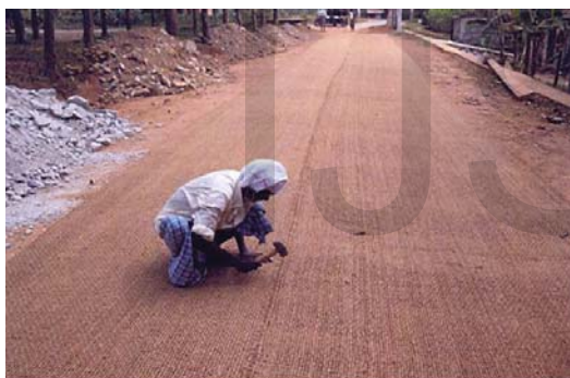
Fixing of Coir Geotextiles to the Road Embankment
