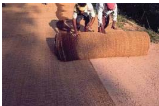
Laying of coir geotextiles in Attukal Pambadi road on 23-09-2011
